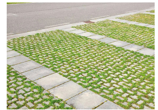
Permeable Paving
