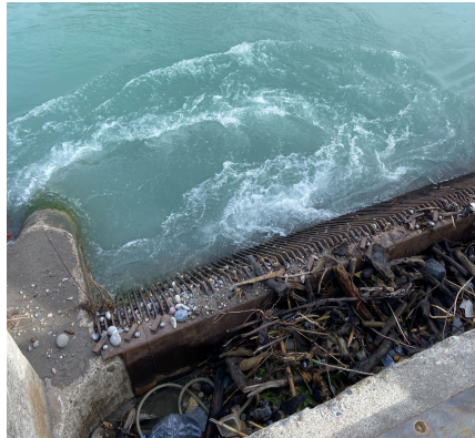
Figure 3: Weir holding back sediment and other debris in the river
